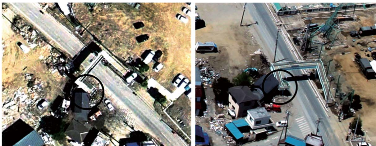
Figure 4. Debris collision observed from satellite image (left) and oblique photographs (right, GSI) after tsunami in Ishinomaki.
