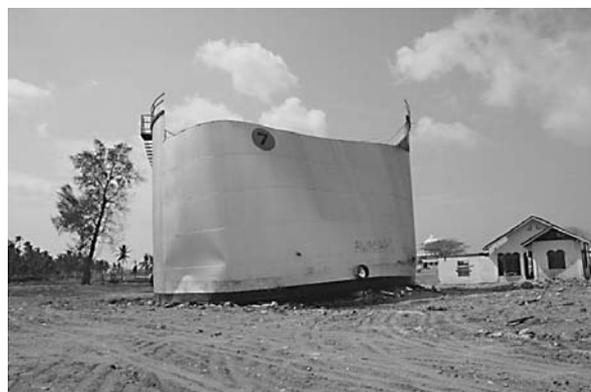
Fig. 12 Relocated oil storage tank at Malahayati
