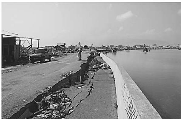
Fig. 9 Failure of river protection walls at Lampulo
