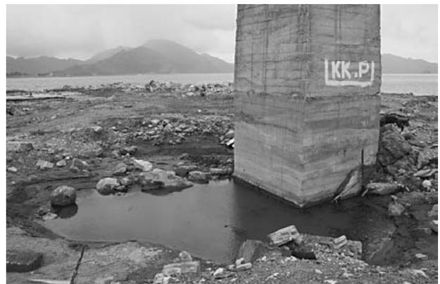
Fig. 5 Erosion behind the monument located at Ulee Lheue
