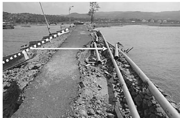
Fig. 11 Minor damage to the embankment for pipelines at Malahayati. Pipelines were dislocated.
