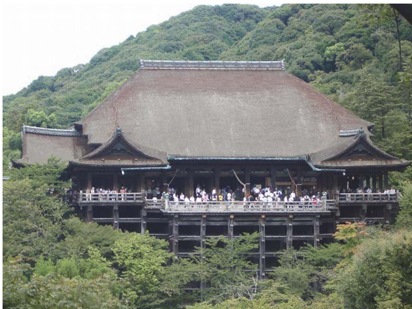
Figure 5. Main wooden structure with stage.
