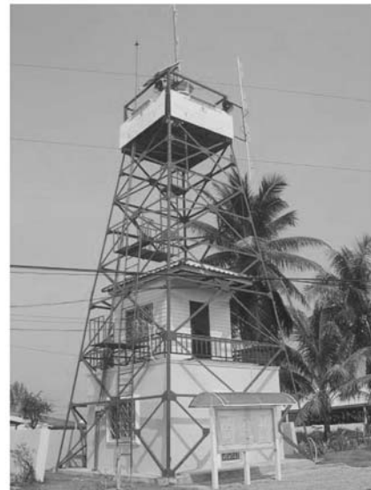
Fig. 10 Dissemination tower at Ban Bang Niang
