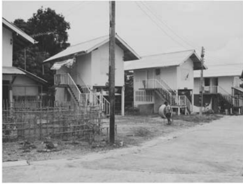
Fig. 19 Construction of permanent houses (Ban Taleanok)
