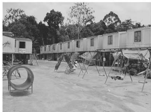
Fig. 16 Temporary house at Khao Lak (Ban Bang Niang)
