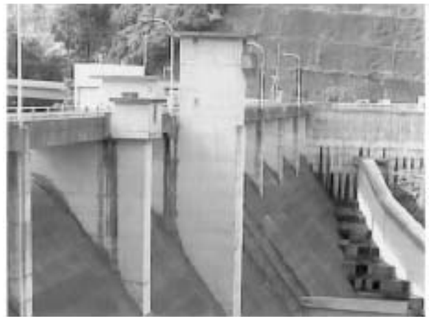
Fig. 3 Downstream views of Kashi Dam from the right bank.
