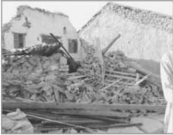
Fig. 7 Damage to a rural house built of stone and timber. Collapse of the roof and failure of the walls produced the major damages to such structures.
